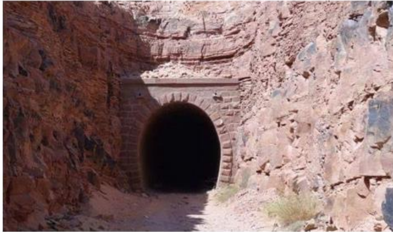
Tunnel crossing of Hijaz Railway, 11
